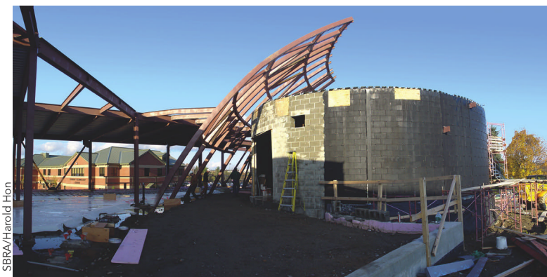
The structural steel frame above the classrooms on the north side of the building is erected and temporarily braces Petal 2 as it cantilevers over the permanent exhibit space.
