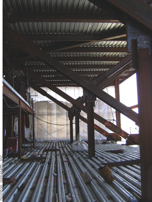
above: Outrigger diagonal braces on the 28th floor.
