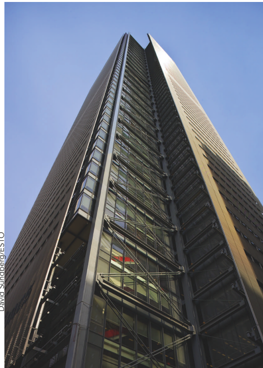
below: Structural elements are brought outside of the building envelope at the four corner notches of the tower.
